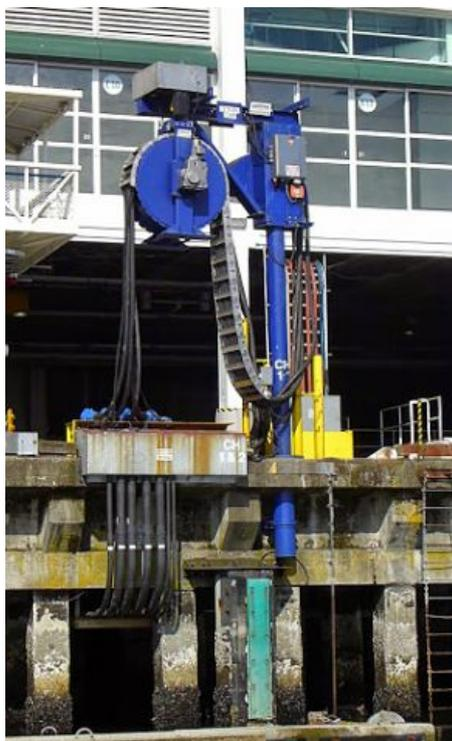
But shore power isn't always plug and play. To make it work in Long Beach, the port had to invest in electric grid trunk lines and substations to bring enough power down to the dock, doubling the price of installing the service to \$190 million.
