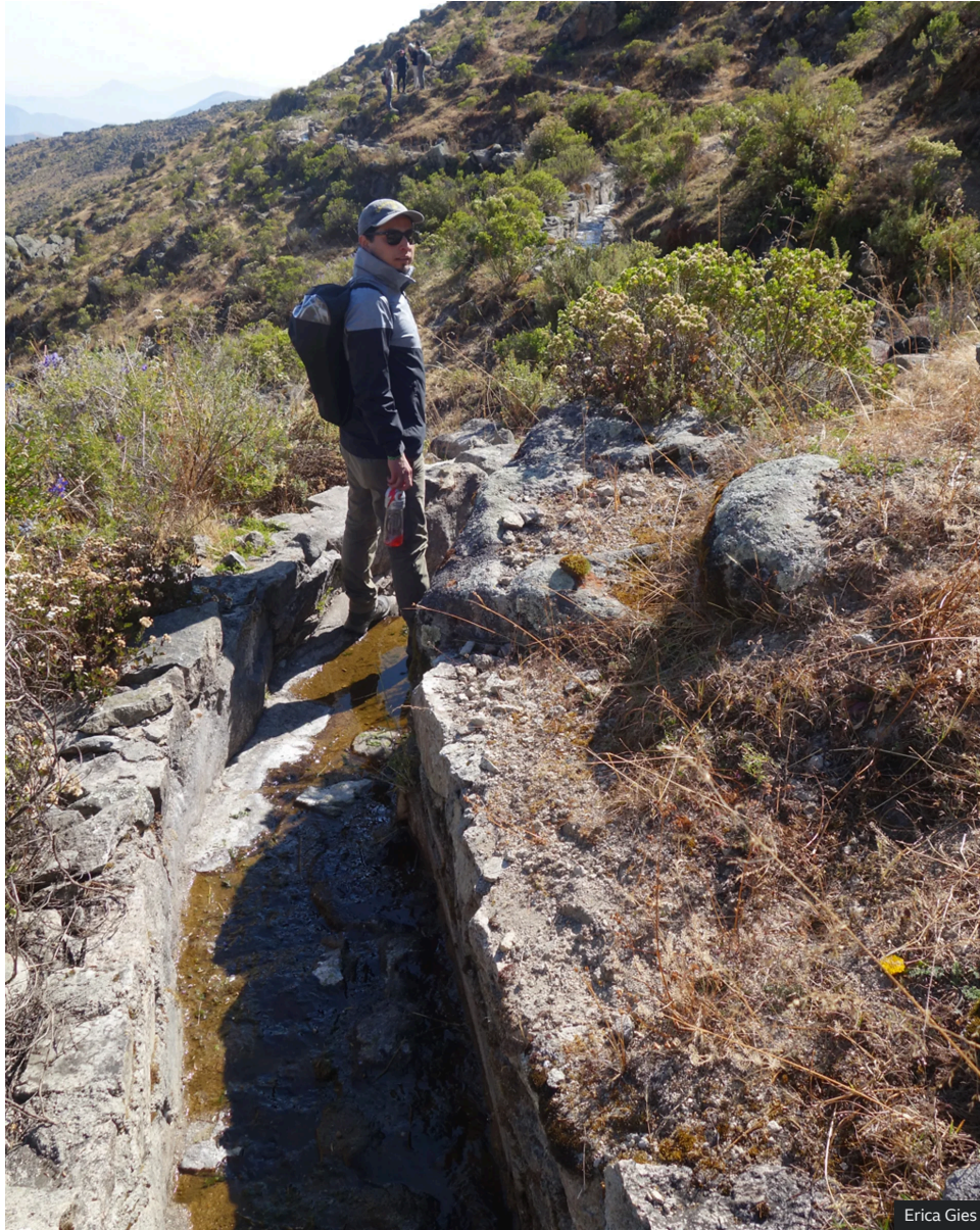
Researcher Boris Ochoa-Tocachi stands in a mortared portion of an amuna, now running low on water, having delivered its flow to the infiltration basins (Credit: Erica Gies)
