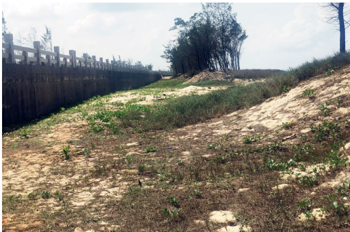
Adaptation to sea-level rise. The Haikou Breathing Sea Wall converts a traditional sea wall into a resilient, permeable barrier against climate change. With terraced planters and revitalized
